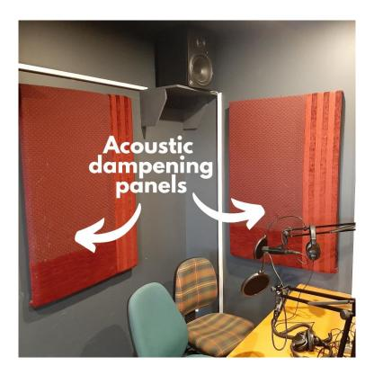
The acoustic panels stop soundwaves from reflecting/bouncing off hard surfaces, thus reducing the 'cavernous room' sounds like echo and reverberation.
